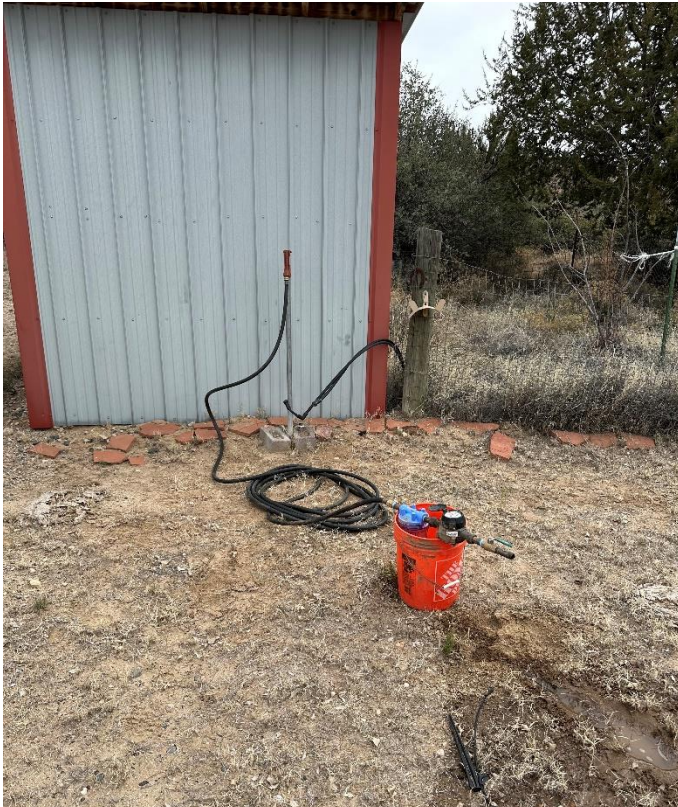
Pump Flow test at yard hydrant
